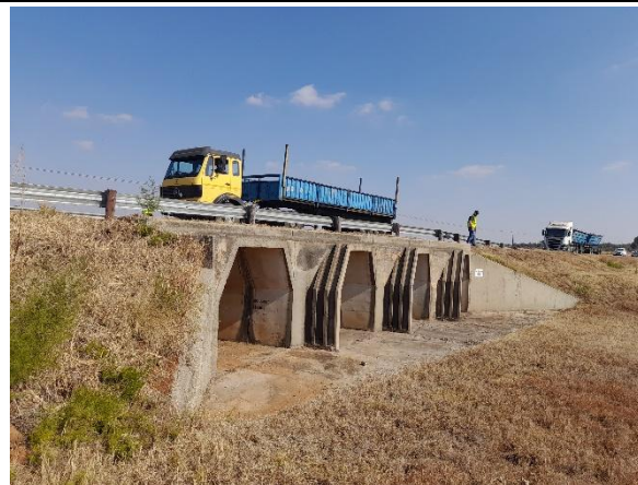
Culvert C4849 at km45.2 to be extended on both sides.
