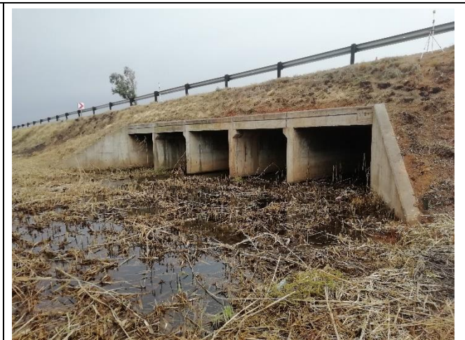
Bridge B5195 at km55.7 at the Schoonspruit River to be extended.
