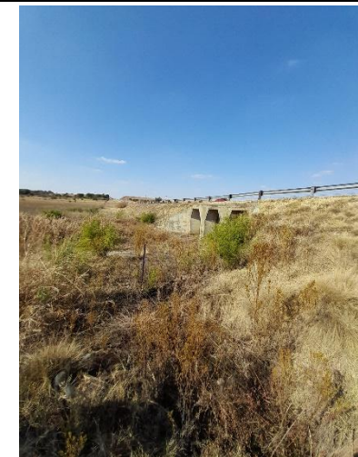
Culvert C4849 at km45.2 to be extended on both sides.
