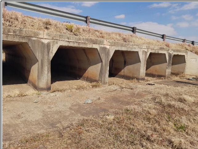
Culvert C4357 at km 8.1 to be extended on both sides with a six cell configuration.
