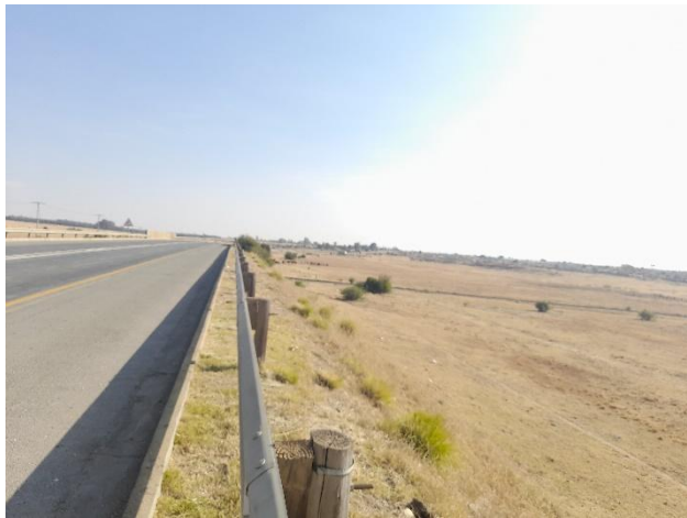
B3552 Coligny Rail Bridge B3552 carries the N14 over a railway line to be widened and rehabilitated.
