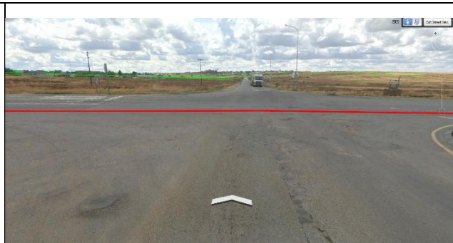
N14/R30 interchange at km54.4 to be upgraded.
