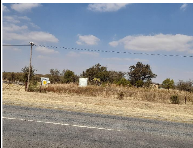
Vegetation to be removed for the increased shoulder width.
