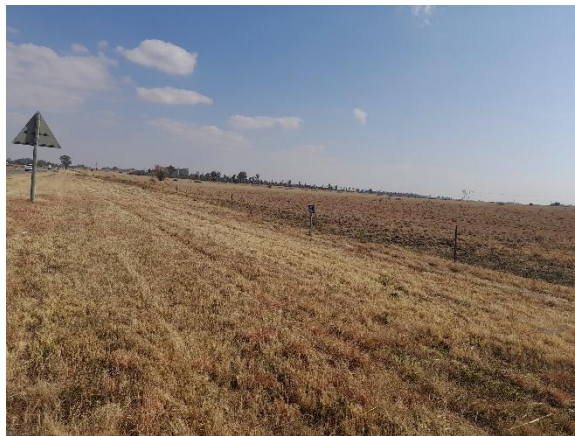
A new culvert with three cells is to be construction at km7.6.
