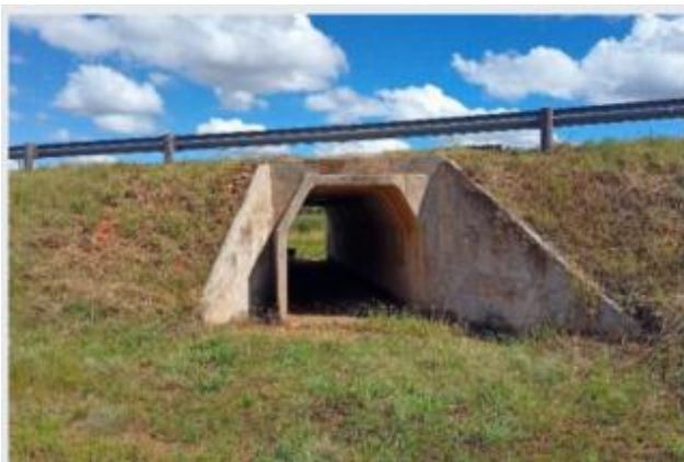
Culvert C4354 at km30.1 to be extended on both sides.
