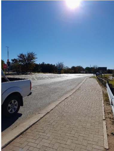
N18 and South Street intersection at Km 47.92 to be upgraded.
