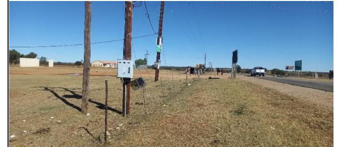
N18 - Section 6 intersection to be upgraded.
