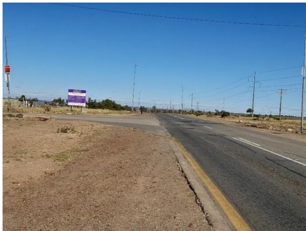
Intersection of N18 and Krish Naidoo Street at Km 45.77 to be upgraded.
