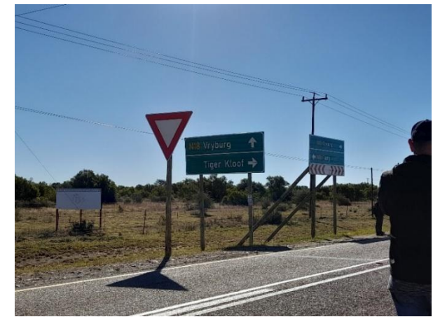
N18 and Tiger Kloof School Access at Km 37.92 to be upgraded.
