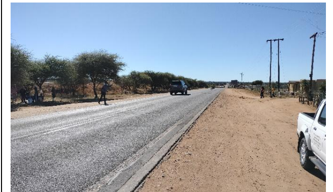
No agricultural practices along the N18 – Section 6 (Tabernacle School Intersection upgrade).
