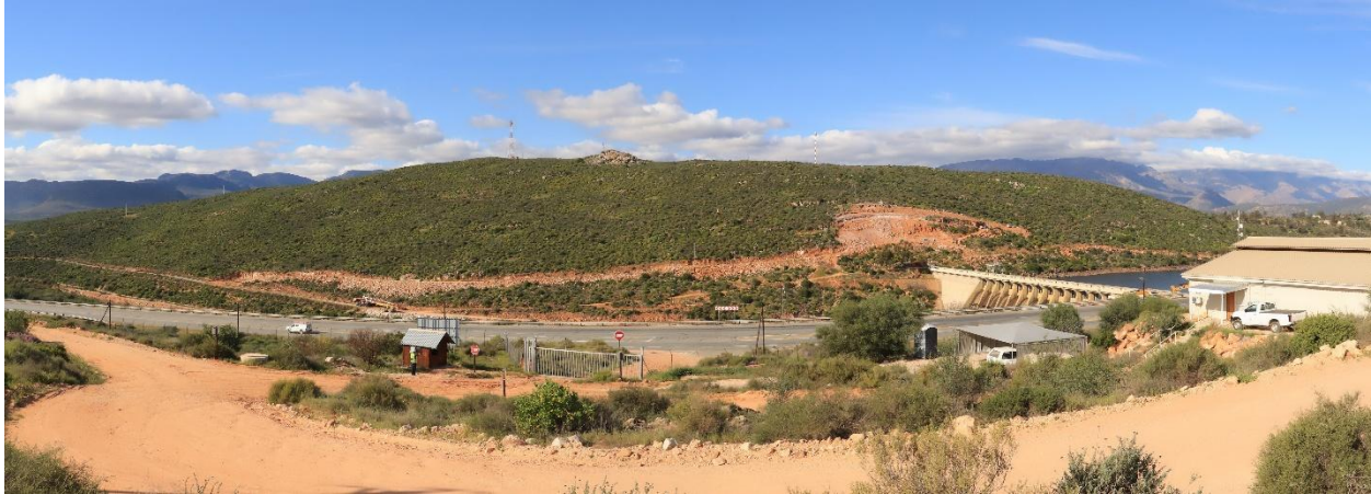
Figure 33: Site photograph illustrating areas of disturbance on the eastern bank associated with the dam wall raising. Note the increased visibility of the road cutting sans vegetative rehabilitation of the road embankment. (Smit, 2025)
