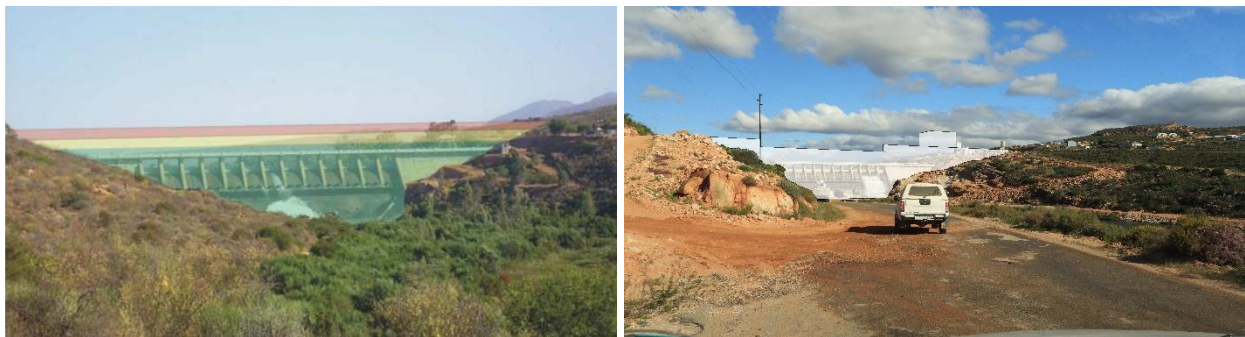
Figure 8: Comparative image of Figure 2 showing a view of the downstream face of the existing dam wall, looking south, illustrating the dam raising alternatives (i.e. green: 5m raising; yellow: 10m raising; red: 15m raising) (Ninham & Shand, 2009 and Smit, 2025)
